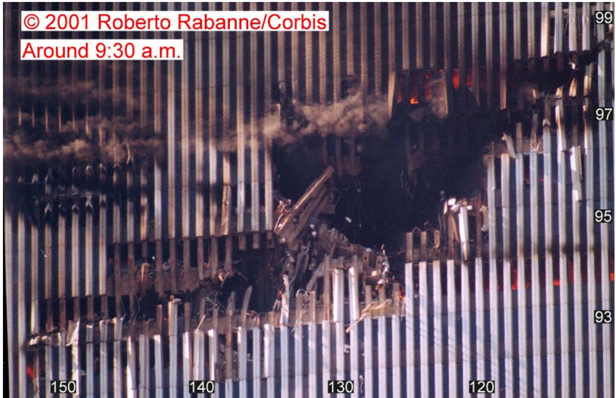
(a) Observed Damage
